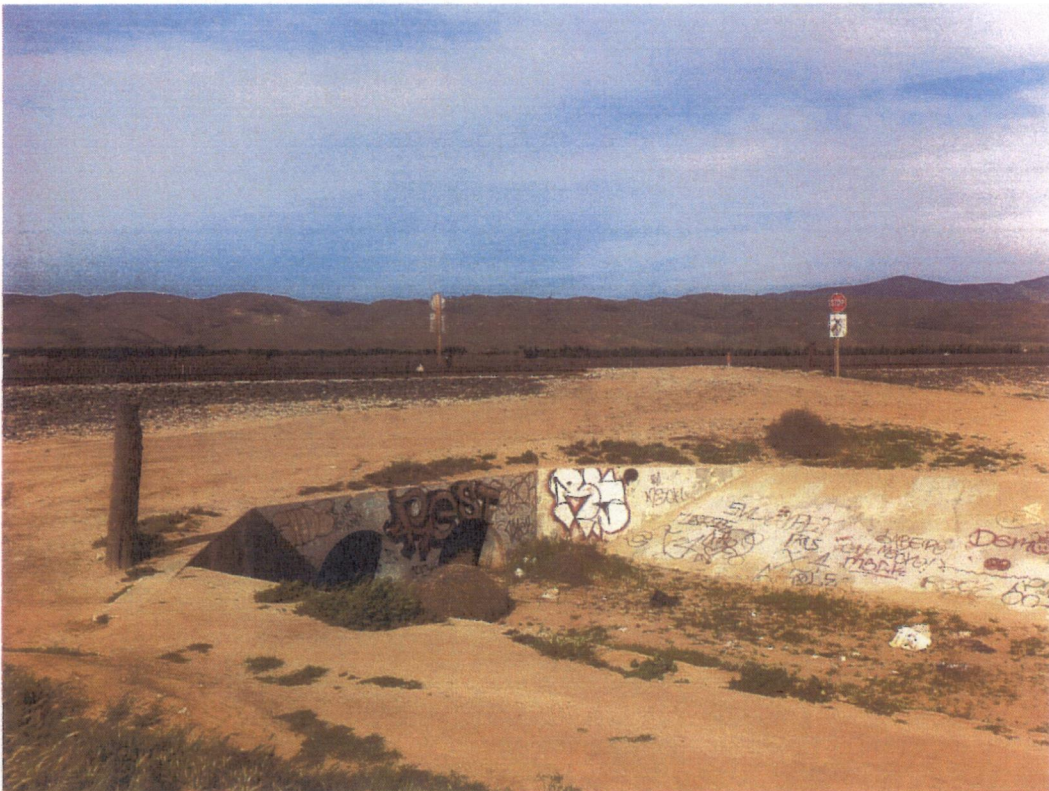
Picture 2: Existing culvert to be replaced with standard concrete bridge
